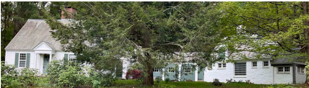
Tree-Shrouded Cow Shed cum White Cottage - Mountain Road
