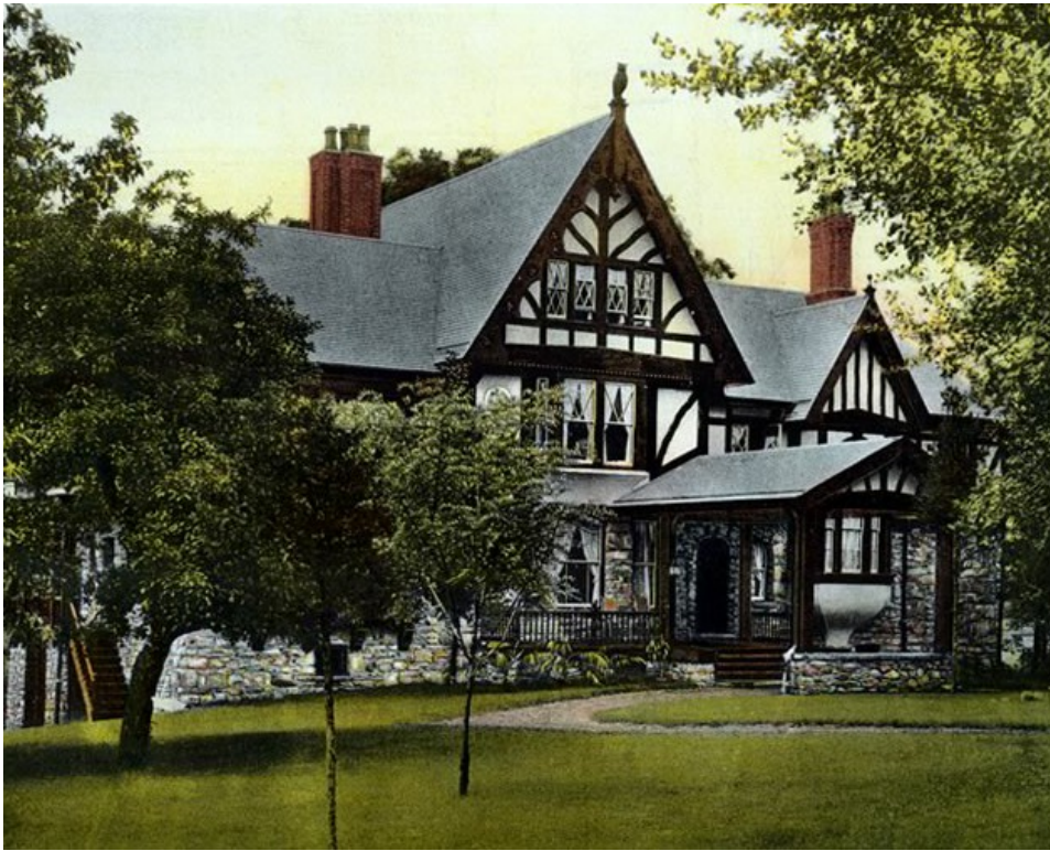
Oak Ridge Cottage (The Owl House) - Bronxville, NY William Winthrop Kent, Architect - 1895
